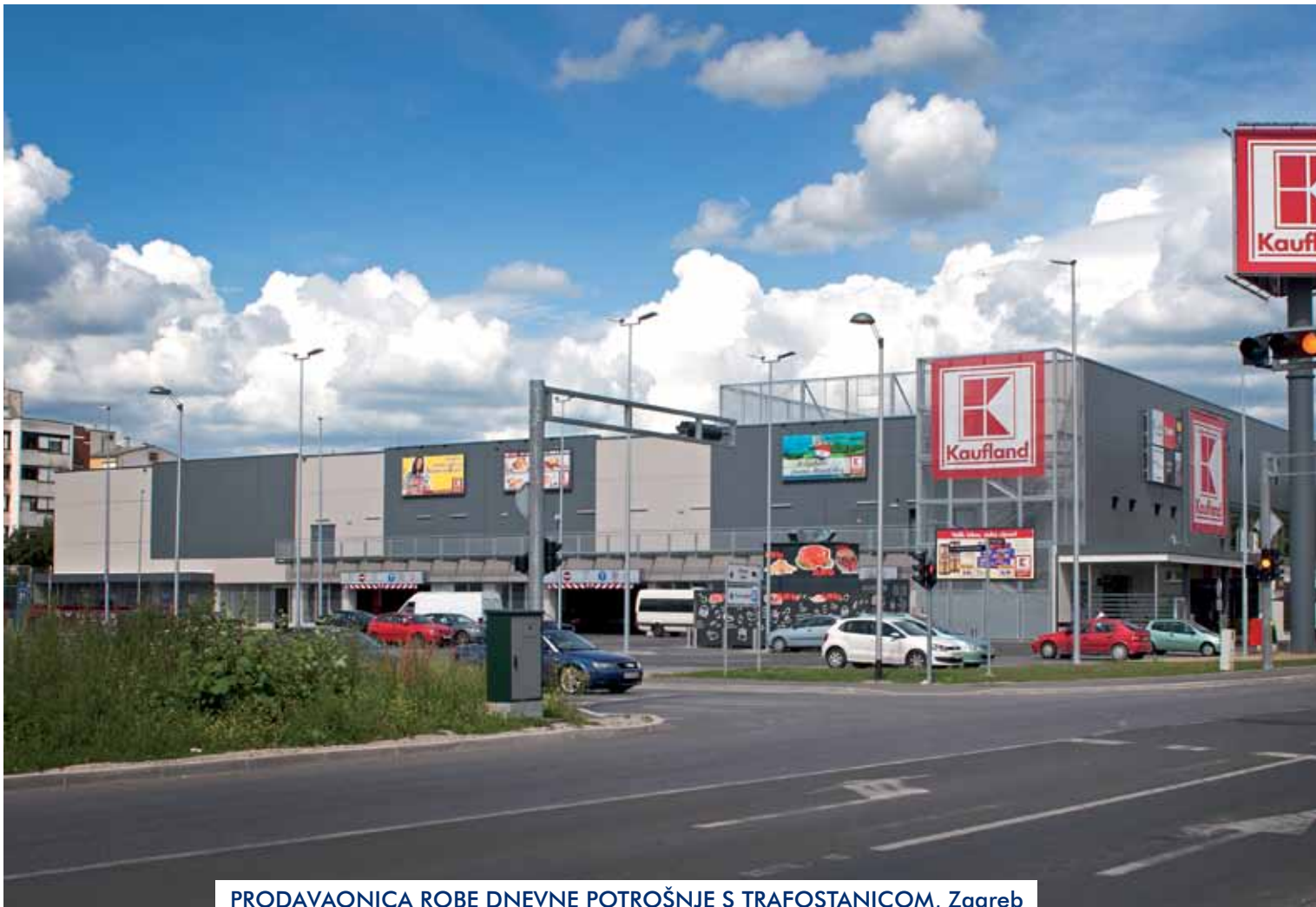
PRODAVAONICA ROBE DNEVNE POTROŠNJE S TRAFOSTANICOM, Zagreb CONSUMER GOODS STORE WITH SUBSTATION, Zagreb
